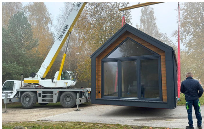
Transfer from semi-trailer to farm trailer using a 35-tonne crane
